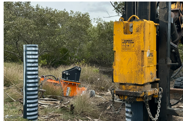
Figure 4. Drop hammer field test on Phill Hill Boardwalk FRP piles
