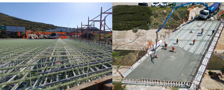
Figure 8. Slab reinforcement with glass fiber bars and casting.
