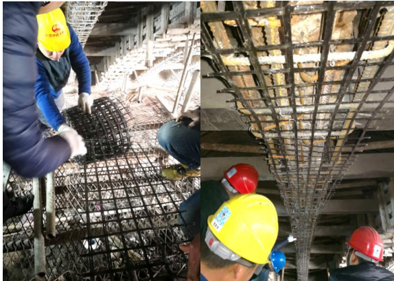
(a) install BFRP grids
