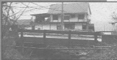
Figure 2: Safe Bridge, Duncan, British Columbia
