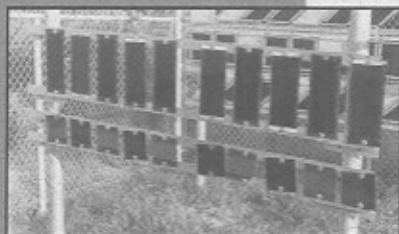
Figure 9: University of Sherbrooke's exposure site for FRP rehab materials.
