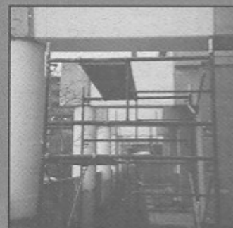
Figure 16: Retrofitting of a specialized structure with FRP
