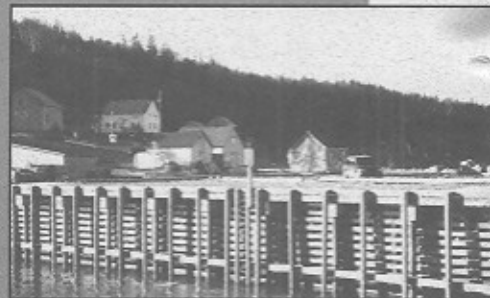
Figure 4: Rehabilitated section of Hall's Harbour wharf
