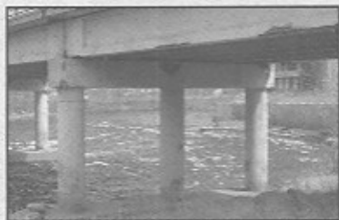
Figure 17: Bridge in Ste-Anne-de-Beaupré, Quebec selected for upcoming laboratory test
