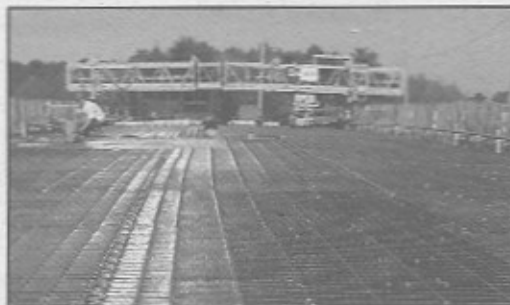
Figure 12: Layout of CFRP grids prior to the final concrete pour
