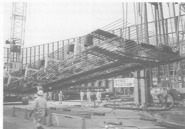
NEFMAC for diaphragm wall at the launching shaft
