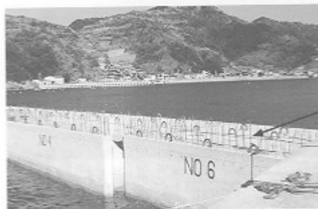
Breakwater caissons overview
