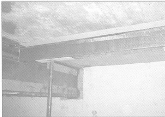
Figure 19: Beam strengthening at Antwerp Zoo.
