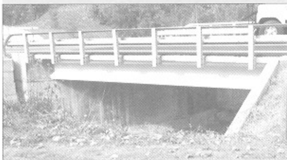
Figure 3: Five-Mile Road Bridge with FRP deck
