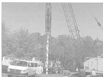
Figure 7: Concrete-filled FRP tubes being driven as load-bearing piles in Florida.
