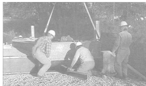
Figure 9: Installation of full-depth FRP bridge.
