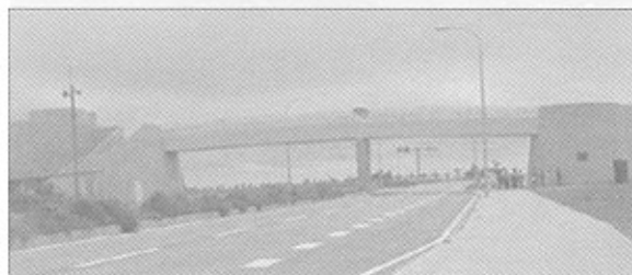
Figure 13: Pedestrian Bridge in Okinawa, Japan.
