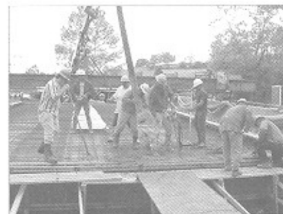
Figure 5: Deployment of CFRP rebars in Two-Mile Creek Bridge
