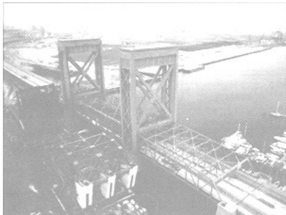
Figure 11: The Schuyler Heim Bridge in Long Beach, California.
