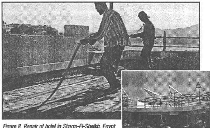
Figure 8. Repair of hotel in Sharm-El-Sheikh, Egypt
