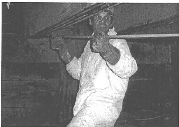
Figure 22: Strengthening of Tourand Creek Bridge.
