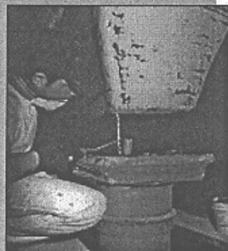
Figure 12: Strengthening of masonry columns with CFRP
