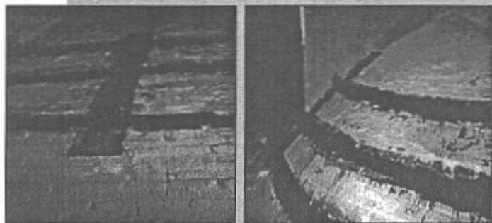
Figure 13: Strengthening of cathedral domes with CFRP.
