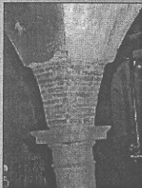
Figure 12: Strengthening of masonry columns with CFRP
