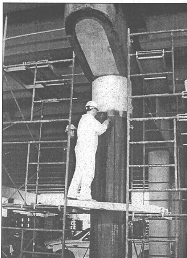
Figure 11: Carbon fiber wrap installation, Minneapolis, Minnesota.
