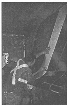
Figure 5: Installation of CFRP sheets.
