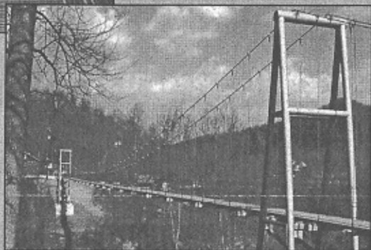
Figure 10: DURAGRID® for deck of suspension bridge in Kentucky.
