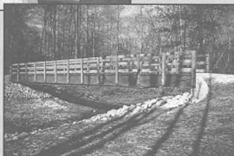
Figure 2: Clear Creek Bridge
