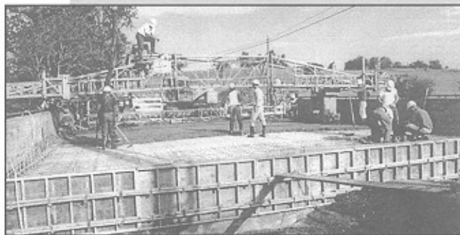
Figure 5: Deployment of GFRP rebars in Roger's Creek Bridge
