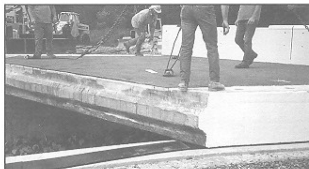
Figure 7: Installation of FRP superstructure
