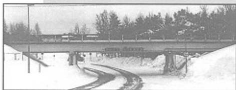
Figure 11: Strengthening of railway bridge in Sweden
