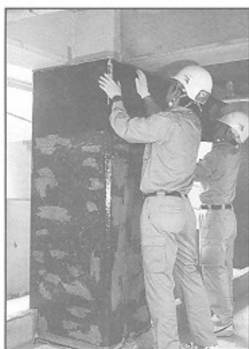
Figure 18: Seismic retrofit of column
