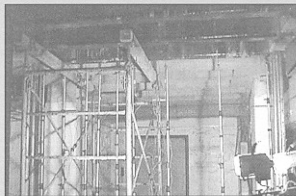
Figure 21: Testing of RC joist strengthened for shear
