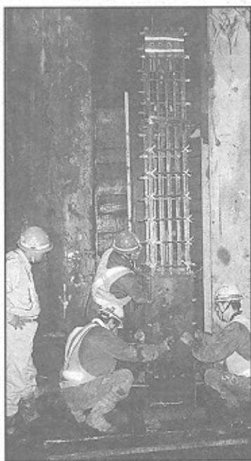
Figure 14. NEFMAC for column reinforcement
