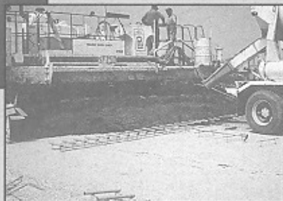
Figure 4. GFRP dowels used in highway in Winnipeg, Manitoba
