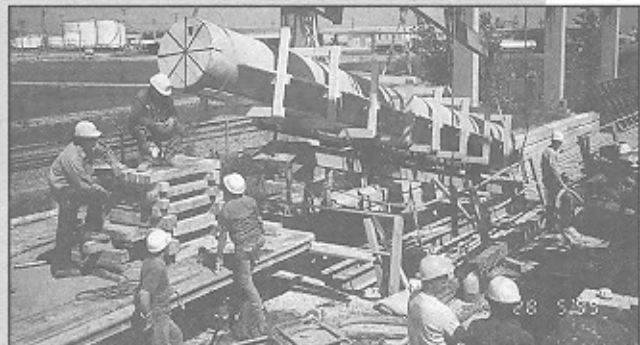
Figure 7. Casting of FRP/concrete hybrid member
