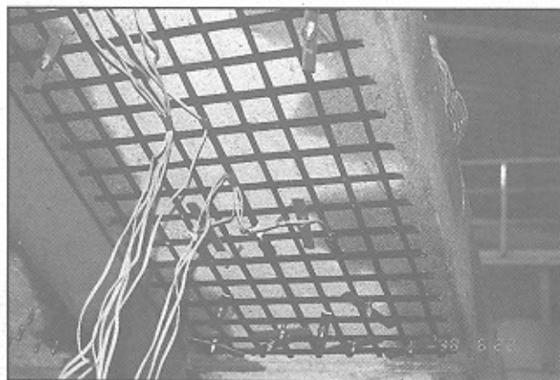
Figure 17. NEFMAC for strengthening RC slabs
