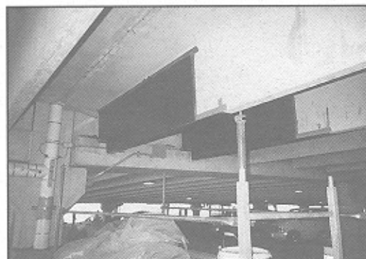
Figure 15. Shear strengthening of prestressed double-tee beams
