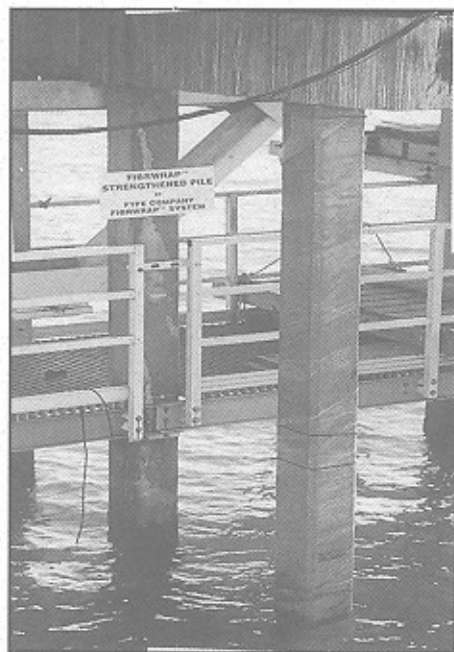
Figure 4. FRP sheets for deteriorated piles
