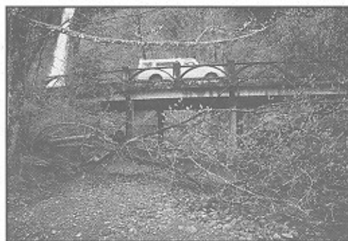
Figure 11. Horsetail Creek Bridge in Oregon, U.S.A.
