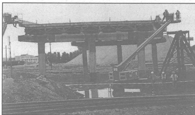
Figure 19. Field testing to evaluate strengthening bridges with FRP
