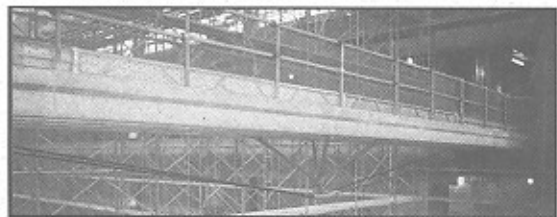
Figure 7. Pedestrian Bridge in Japan
