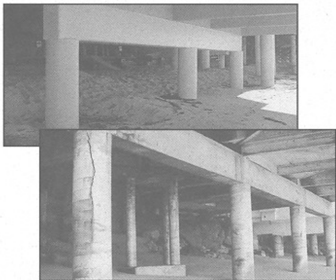
Figure 10. Rehabilitation of Continuous Beam and Column in Malibu, California
