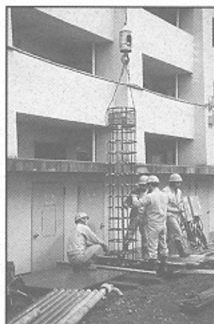
Figure 8. NEFMAC Mesh for Temporary Piles
