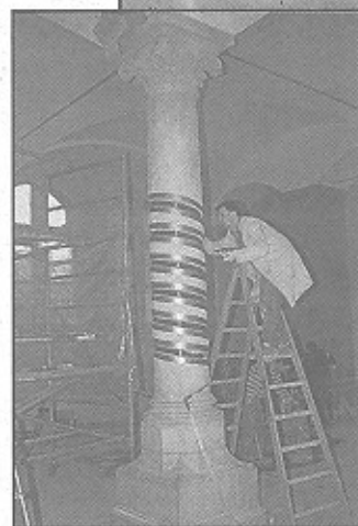
Figure 4. Strengthening of a Limestone Column
