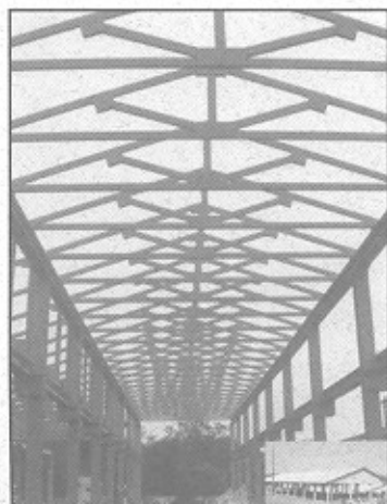
Figure 13. FRP structural systems for sheep barn.
