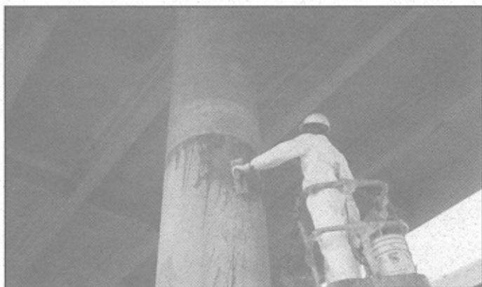
Figure 12. Repair of Interstate Highway 40 in Oklahoma City.
