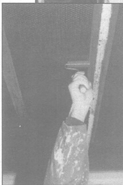
Figure 6. Strengthening of Greenbridge Subway in the United Kingdom.
