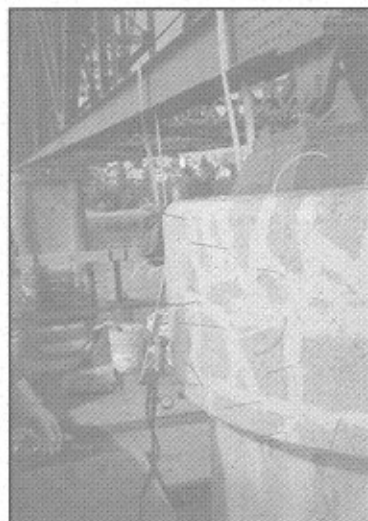
Figure 6. Epoxy Injection of the Pier Cap Prior to Strengthening.
