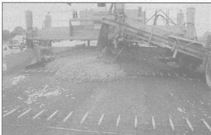
Figure 2. Assembled GFRP Dowels Before Casting of Concrete.
