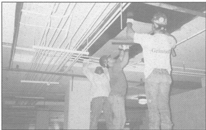
Figure 8. Installation of CFRP Sheets Without Interference with Existing Mechanical System.
