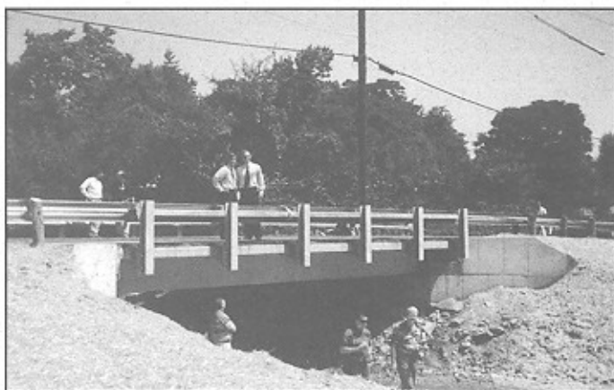
Figure 8. GFRP Bridge Monitored by Optic Sensors, Ohio, U.S.A.
