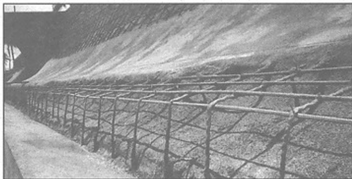
Figure 14. L-Shaped C-Bar Dowels for the Seawall
