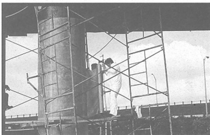
Figure 7. Rehabilitation of Champlain Bridge, Montreal, Canada
