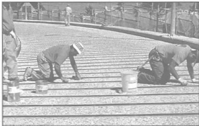
Figure 8. Ferry Bridge Horgen, Switzerland
