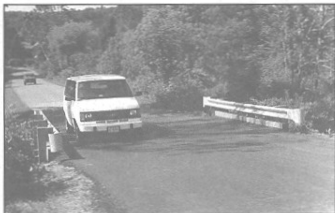
Figure 9. Composite Beams for Tom's Creek Bridge, Blacksburg, Virginia
