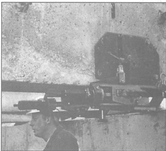
Figure 14. Prestressing of CFRP Plates Bonded to Concrete Beams
