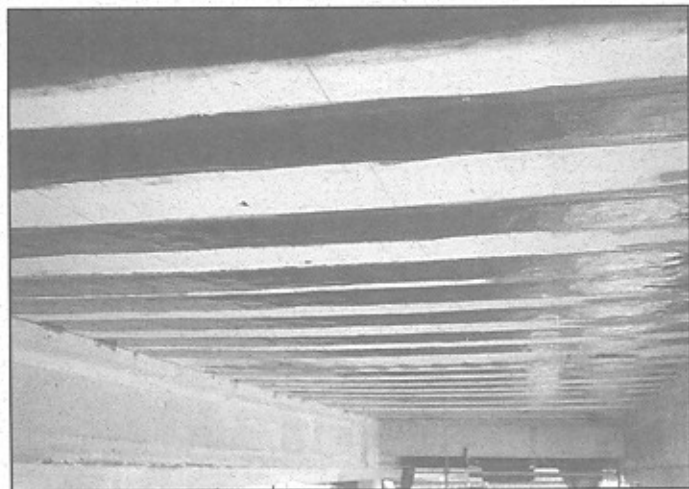
Figure 11. Repair of a Swimming Pool in Belgium
