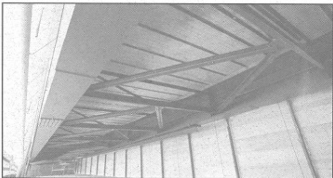
Figure 9. Strengthening of Oberriet Bridge.
