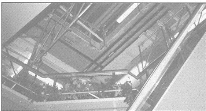
Figure 3. Strengthening of City Shopping Centre, Winterthur, Switzerland.
