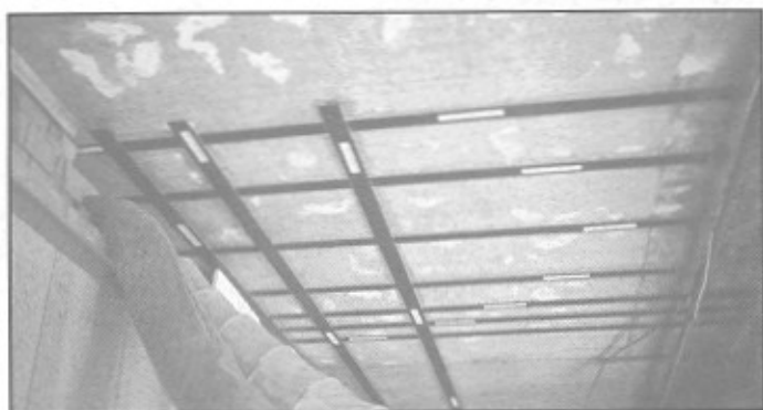
Figure 4. Strengthening of Two-way Slab.
