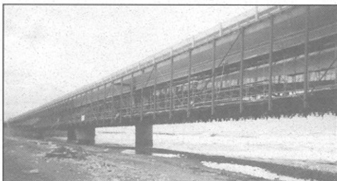
Figure 2. Repair of Highway Bridge.
