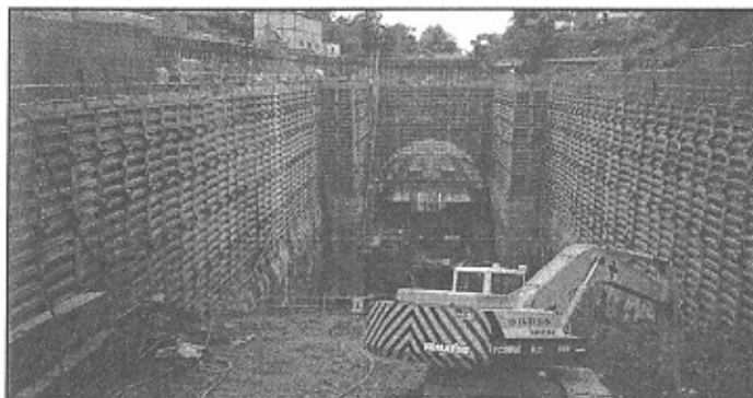
Figure 2. FIBRA ground anchors for temporary wall.
