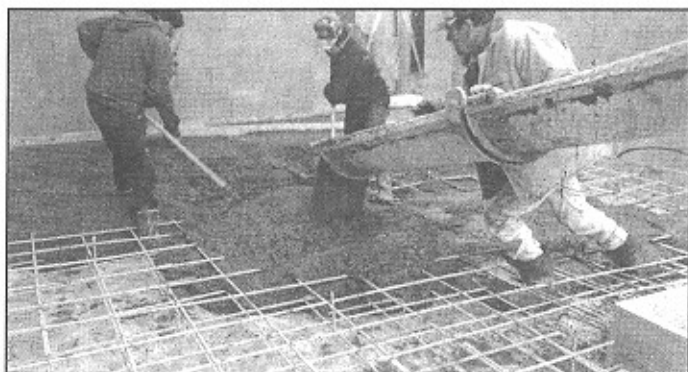
Figure 1. GFRP reinforcement for MRI floor.
