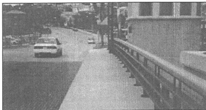
Figure 11. SAFEPLATE™ fiberglass panels for sidewalk.
