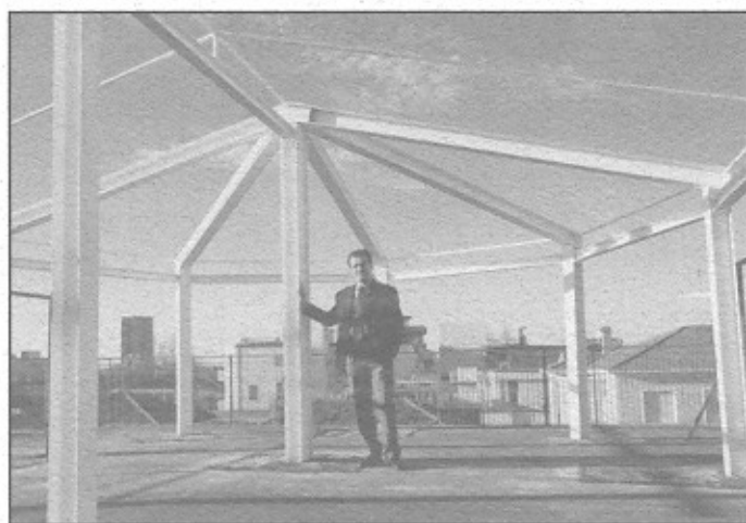
Figure 7. GFRP for floor terrace, Rimini, Italy.
