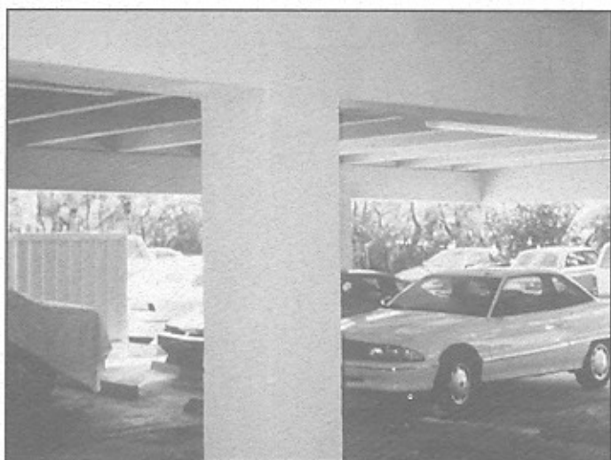
Figure 2. The main beam after completion of the repair.
