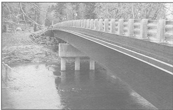
Figure 3. Clallam Bay, Washington, using FiRP™ glulams girders.
