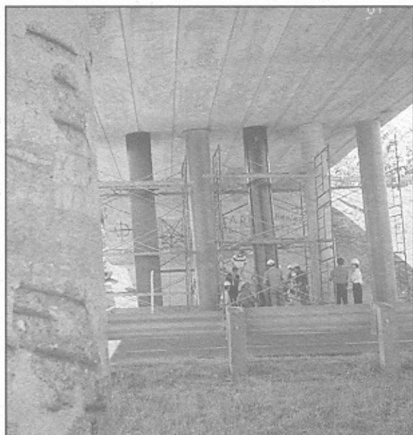
Figure 6. Rehabilitation of Highway 10 overpass in Canada.
