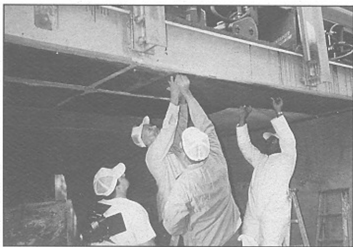
Figure 4.0 Carbon Fiber Plates for Ohio Bridge
