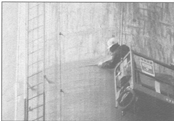
Figure 6. Repair Work for Deteriorated Chimney
