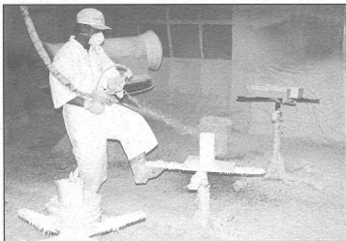
Figure 5. Sprayed Fibre Reinforced Plastic for Repair
