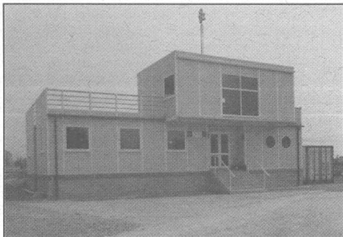
Figure 10. Advanced Composite Site Office Building.
