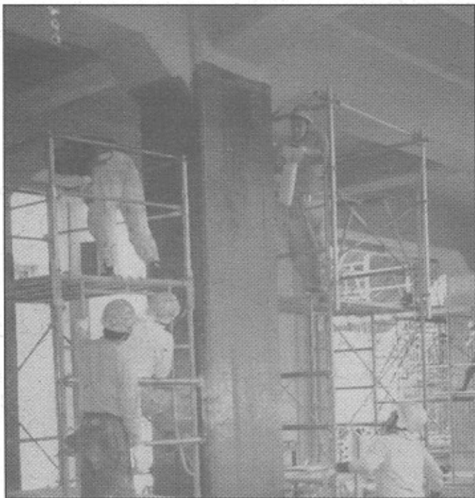
Figure 7. Rehabilitation using CF Sheets.
