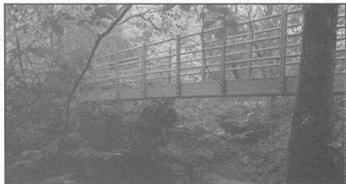
Figure 9. Shank Castle Footbridge.
