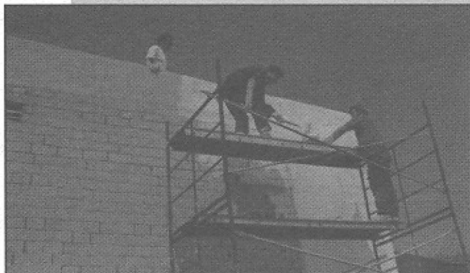
Figure 2. Application of composite fabrics to the URM wall (Courtesy of Structural Rehabilitation Corporation)
