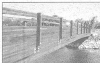
Figure 11. Taylor Lake Bridge, The Dalles, Oregon
