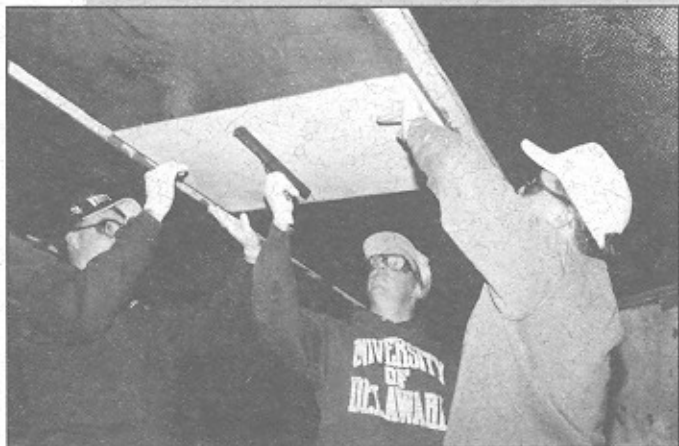
Figure 7. Rehabilitation of Foulk Bridge #26 Wilmington, Delaware
