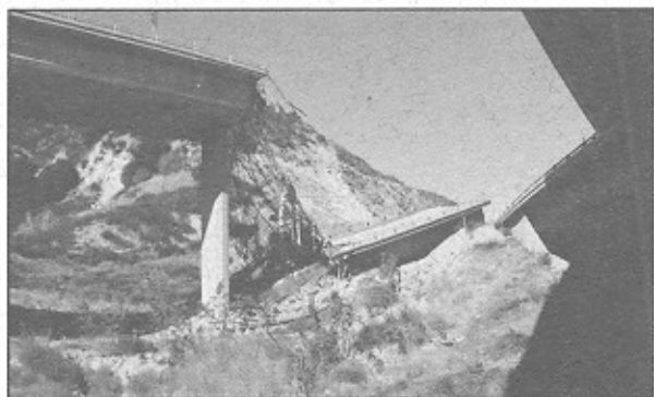
Figure 4. Bridge failure during Northridge Earthquake in California
