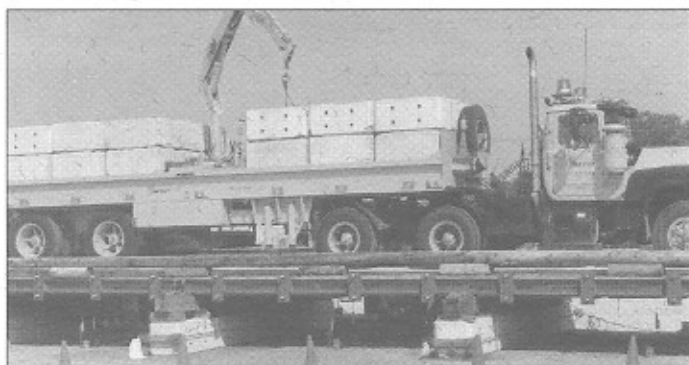
Fig. 2. Proof test of the prestressed log bridge
