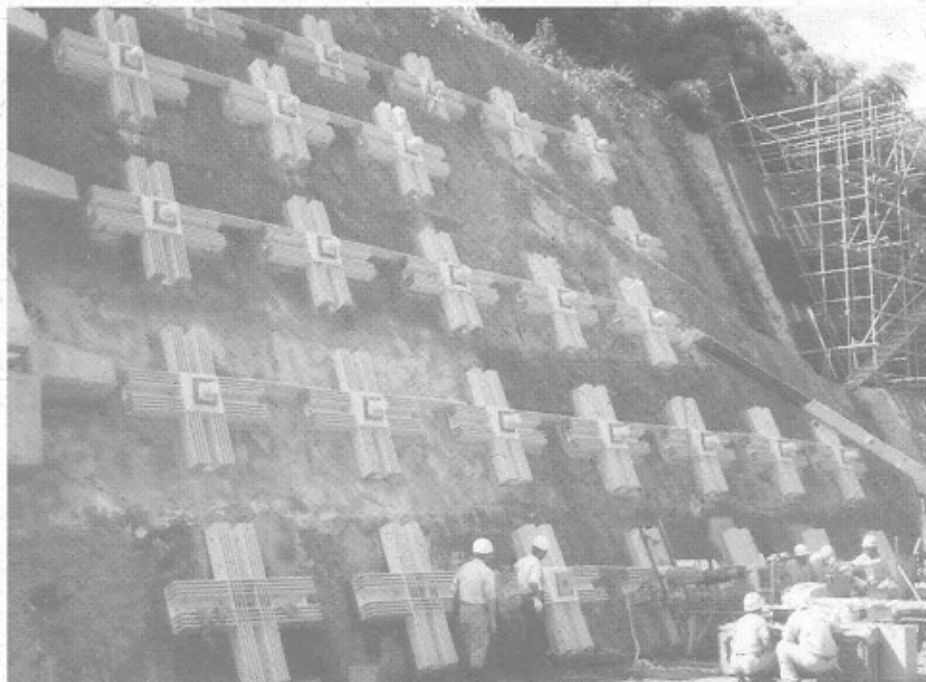
Fig. 5. Ultra-light ground anchor using Aramid FRP
