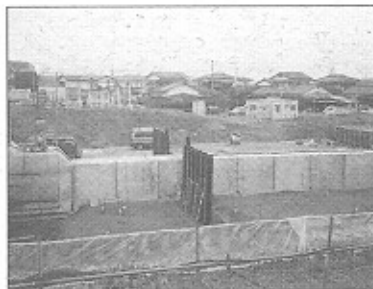
Figure 3. Flexible Box-culvert drainage system, Ariake, Japan
