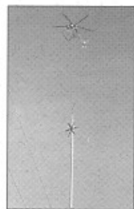
Figure 5 Helicopter installation of Composite Electric Pole
