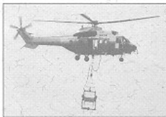
Figure 7a. Helicopter guiding Aramid pilot rope
