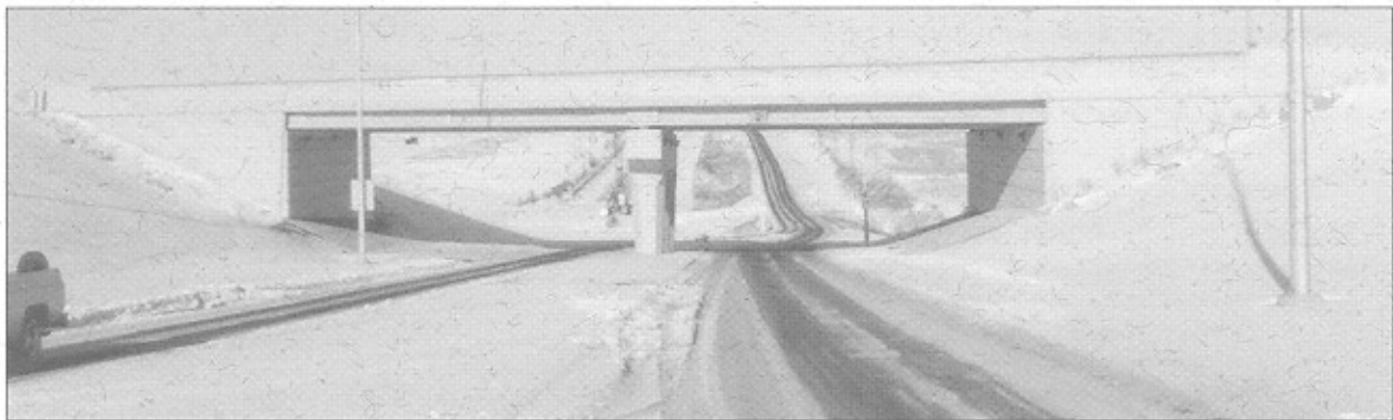
Figure 11. Beddington Trail/Centre Street Bridge, Calgary, Canada
