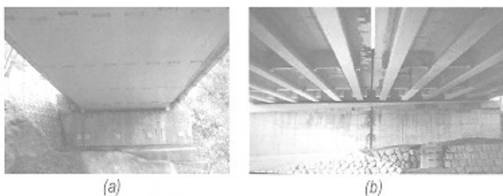
Fig. 2 Strengthening of: (a) a hollow-slab bridge at a National Route; and (b) a post-tensioned T-girder highway bridge with the P-PUT
