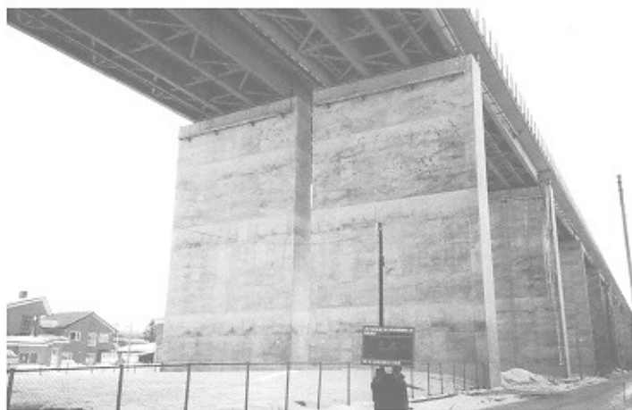
Fig. 4 The Chitosegawa Bridge strengthened with AWS method
