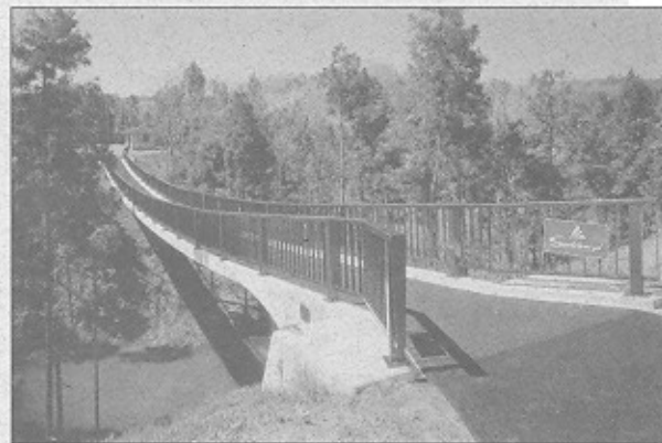
Figure 2. Birdie Bridge in Southern Yard Country Club, Ibaragi
