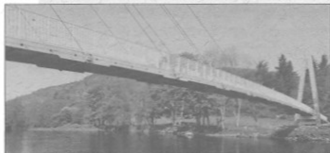
Figure 1. Linksleader Footbridge, Aberfeldy Golf Club, Scotland
