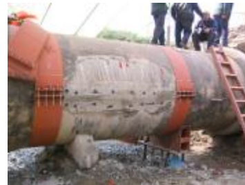
Crack completely sealed.
