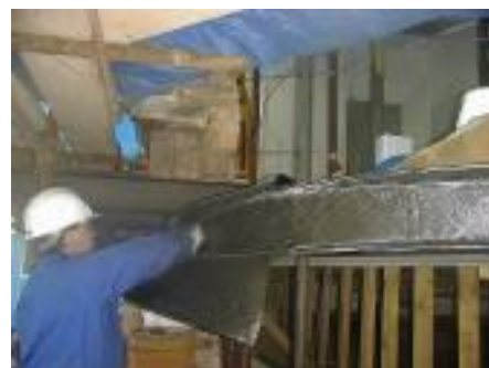
Cast Iron Beam.
