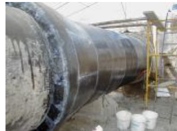
Strengthened Pipe with Tyfo SCH-41 Carbon System.
