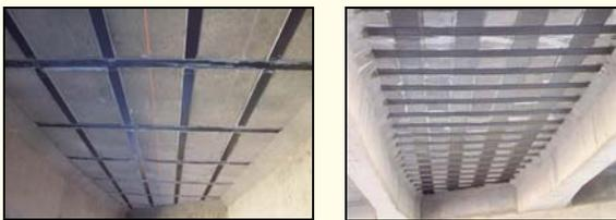
**Figure 3. Completed Rehabilitation, Adhesive Bonding (Left) and Wet Lay-up (Right)**
