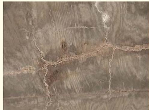
Figure 2. Transverse and Longitudinal Cracking on Bridge Deck
