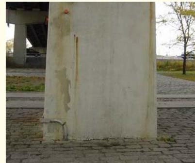
**Figure 10(a). E-Glass FRP Wrapped Column**
