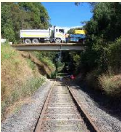
Fig. 4: 18 m Bridge Girder Installed
