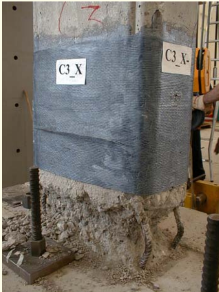
Fig. 3: Concrete crushing, and rebar buckling are combined with fracture of the FRP jacket at the base of the column.
