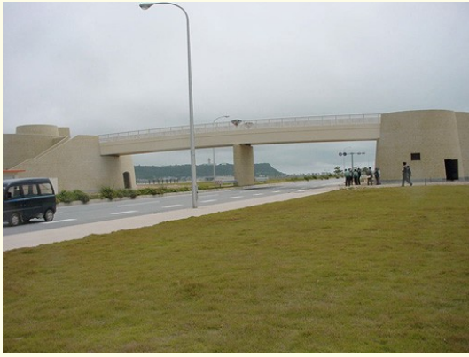
Fig. 4: The Pedestrian Bridge in the Road-Park of Ikei-Tairagawa in Okinawa
