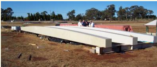
Fig 3: 18m Bridge Girders Before Shipping to Site
