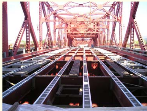
Fig. 3: The Bridge's longitudinal stringers were prepared for placement of FRP panels.
