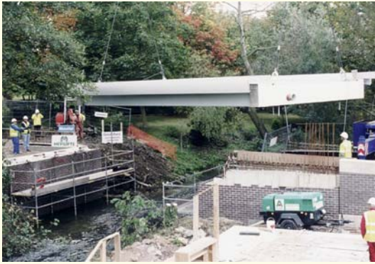
Fig. 3: GFRP West Mill Bridge in construction using ASSET system
