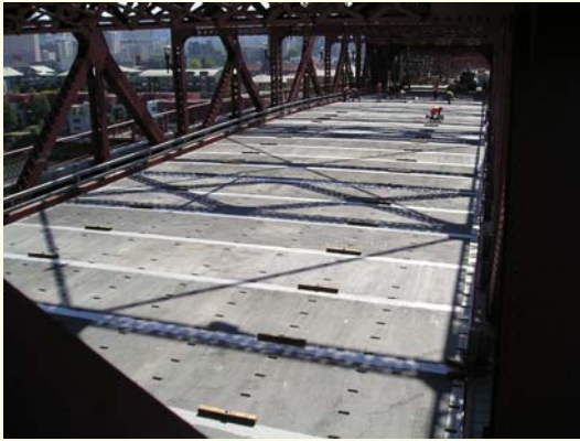
Fig. 6: All FRP panels were in place after two shifts.
