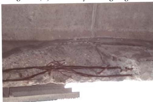
Figure 3(b) – Significant Loss of Concrete and Damage to Steel Reinforcement
