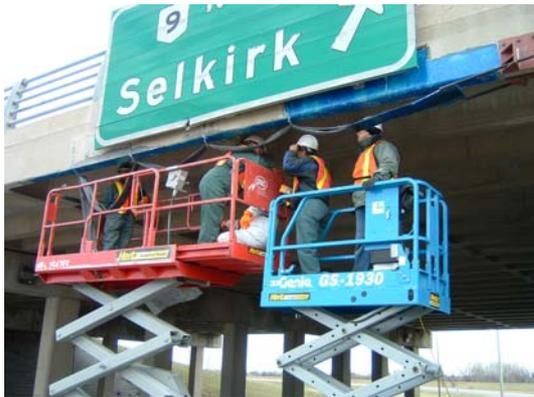
Figure 6 – Placing the CFRP Sheets
