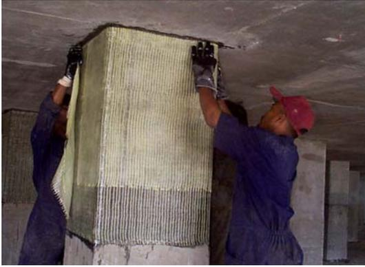
*Figure 2: Seismic retrofit of supporting columns for a cryogenic tank in Gujarat, India<sup>2</sup>*
