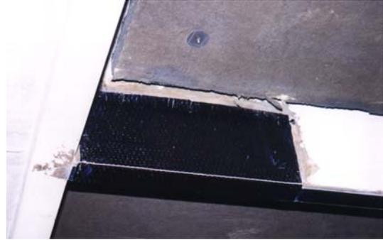
*Figure 5: Wet Layup System Used to Anchor Adhesively Bonded Prefabricated Strips in the Saddle Dome*
