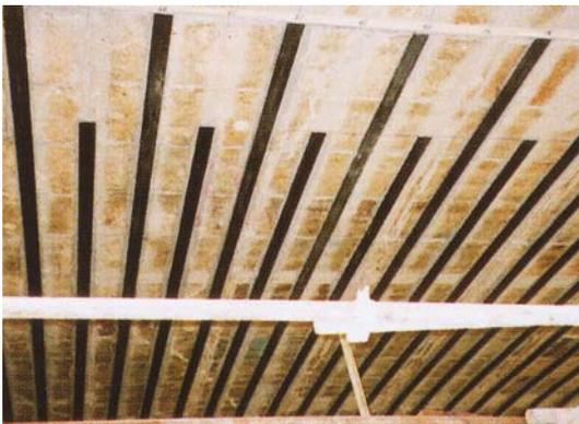
*Figure 3: Strengthening of slab in a shop house, to take heavy computer networking equipment, in Malaysia<sup>3</sup>*
