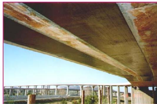
*Figure 1: Flexural strengthening of a highway RC bridge slab in China<sup>1</sup>*
