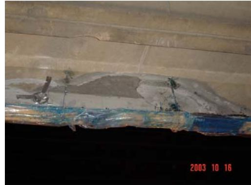
Figure 7 – Plastic Sheets to Maintain the Curing Conditions
