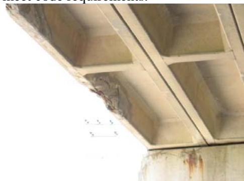
Figure 3(a) – Severely damaged girder
