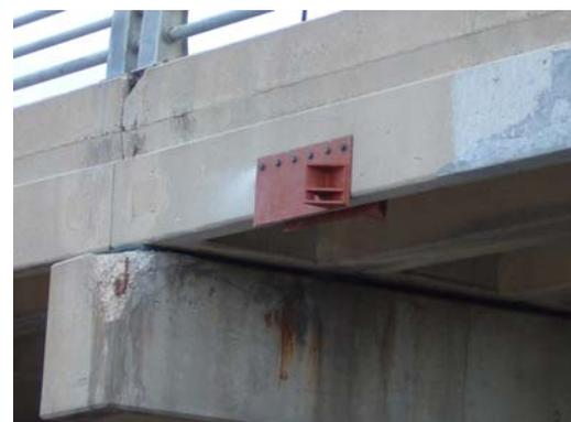
*Figure 5: Mounting of Shear Plates*
