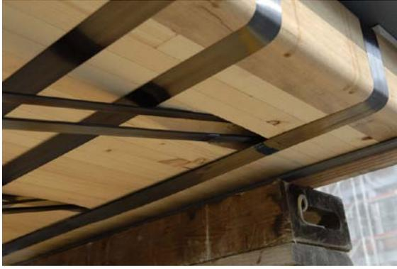
Figure 6. Bowstring, composed of non-laminated thermoplastic CFRP strap elements, going through the hole in the glulam deck to the termination of the pin-loaded strap. The stiffness EA of each bowstring is 18 MN. The stiffness of the lateral tendons is 3 MN
