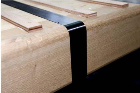
Figure 9. Top: The wooden spacers should avoid rottenness of the glulam under the GFRP plate
