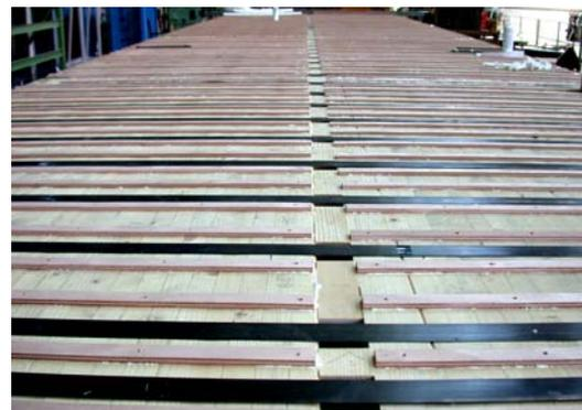
Figure 3. Bridge deck after lateral post-tensioning. The location of the original gap is in the centre of the photograph still visible. The wooden spacers should avoid rotteness of the glulam under the GFRP plate
