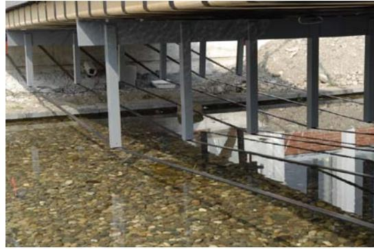
Figure 10. Bridge with CFRP bowstrings after installation
