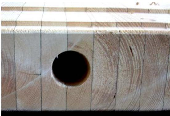
Figure 2. End of the glulam plate. Overall depth: 16 cm. The cuts on top enable to fit with the GFRP cross beam as shown in Figures 7 and 8. The hole of 60 mm diameter is leading to the termination of a bowstring
