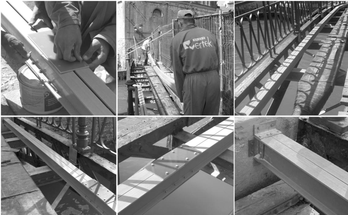
Figure 4. Installation phase of GFRP pultruded profile
