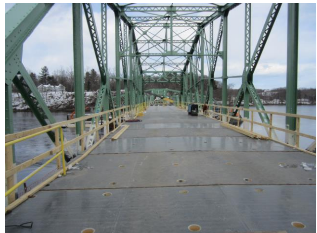
Continuous transverse FRP deck on new steel girders.
