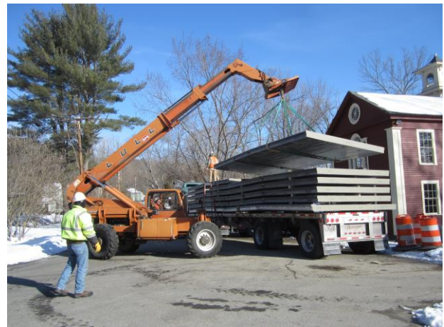
FRP deck panels delivered to jobsite.
