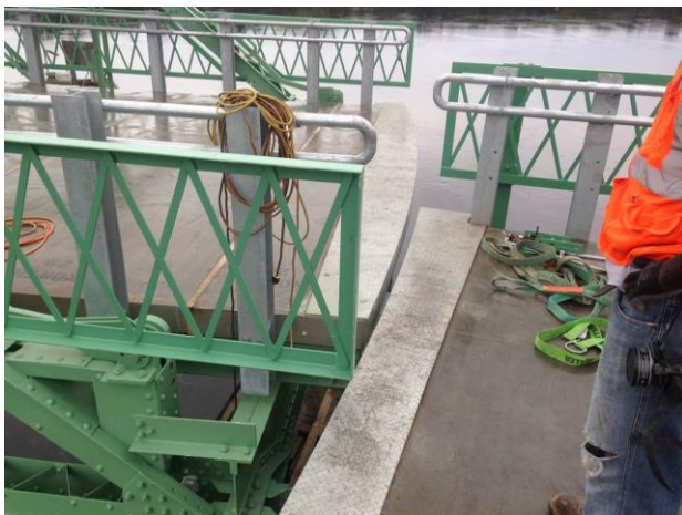
Deck panels fabricated to accommodate swing span.
