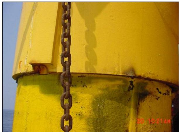
Fig. 1 Traditional welded metal clamp repair [11]
