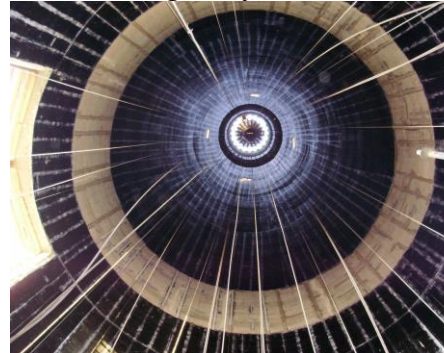
Seismic Strengthening of Concrete Chimney using FRP
